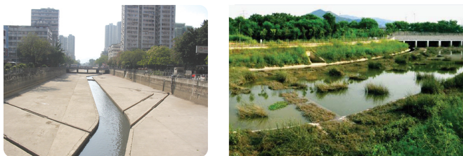
Figure 2. Concrete lined drainage channel (left) Biodiversity-friendly drainage channel (right)
